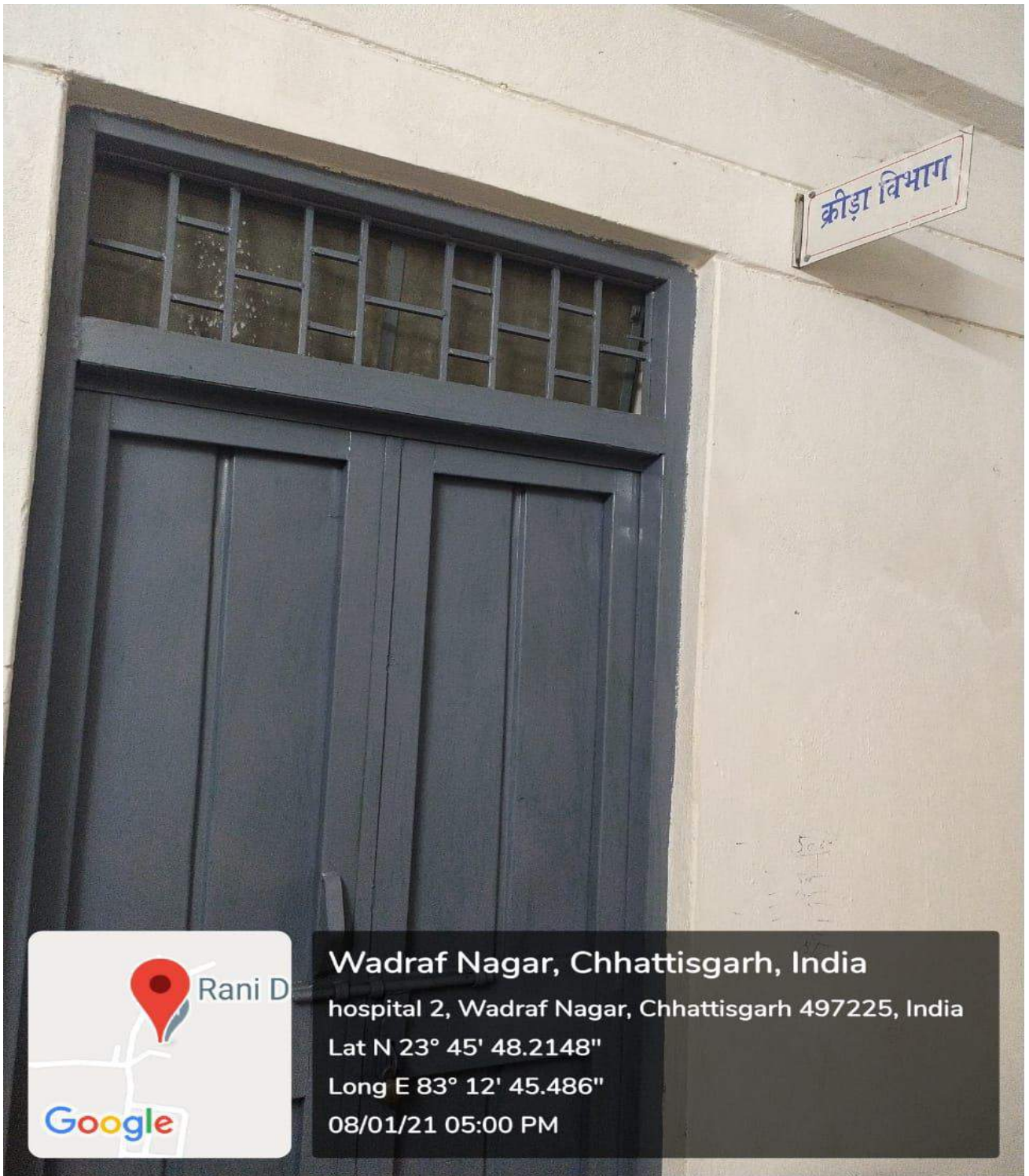
GEO TAGGED PHOTO OF SPORTS ROOM ENTRY GATE
